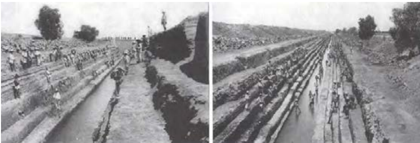
Constructing the Great Drainage Canal, ca. 1890
